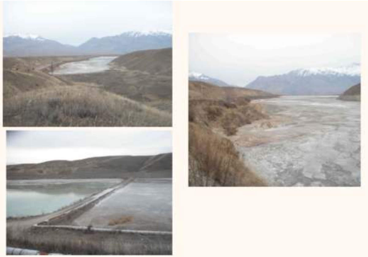
Various views of Makmal gold tailings dam
