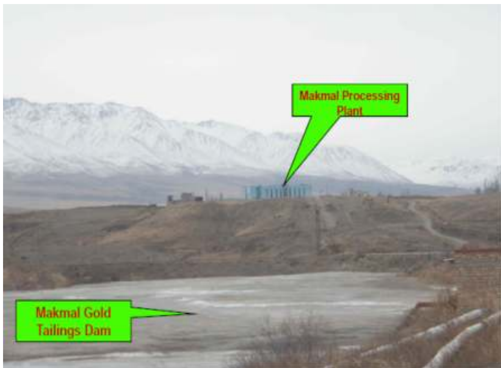
Makmal gold tailings dam ( foreground ).
