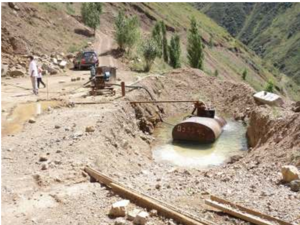
Kuranjayloo – water reservoir for drilling & dewatering adits
